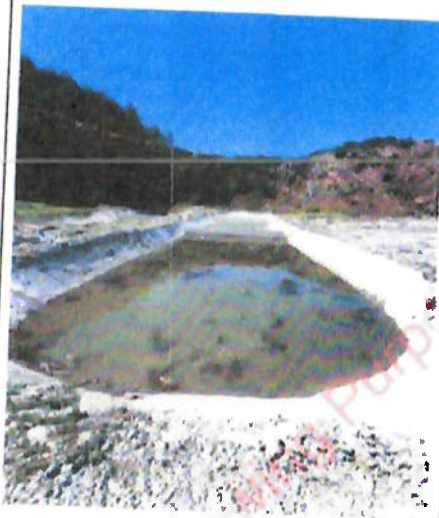
(b) Secondary Pond Tank System in South-western corner of the site. Long Linear concrete lined Ponds with baffle walls.
